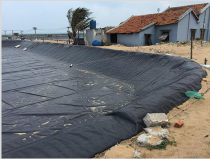
A lined pond along the coast in the South of Vietnam. This was brand new and constructed in response to EMS (AHPNS).
